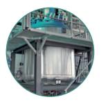
A cascade control system of the cooling towers allows us to save 54.5% in kW, which is equivalent to the non-emission of around 1,370 kg of CO<sub>2</sub> per month
